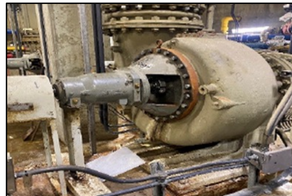
Chesterton 442 Split Seal resulted in increased reliability and a reduction in flush water usage.
